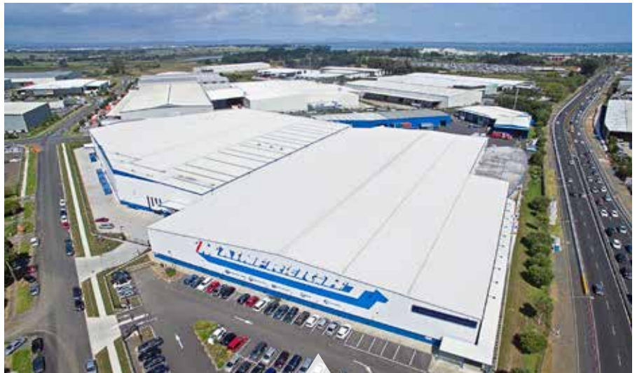
Our investment in the extension for our specialist food grade temperature controlled Westney Road Warehouse where our team is led by Travis Hari
