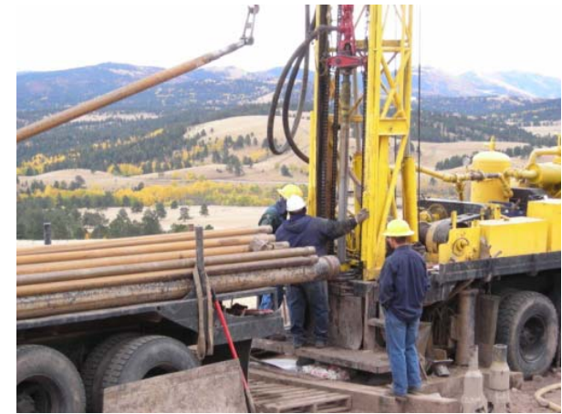
Drilling at the Taylor Ranch Uranium Project.
