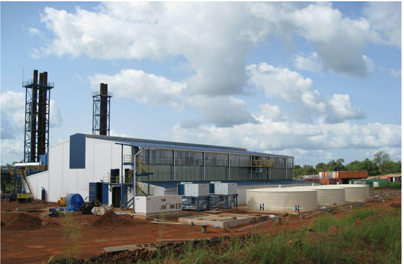
Power station construction completed
