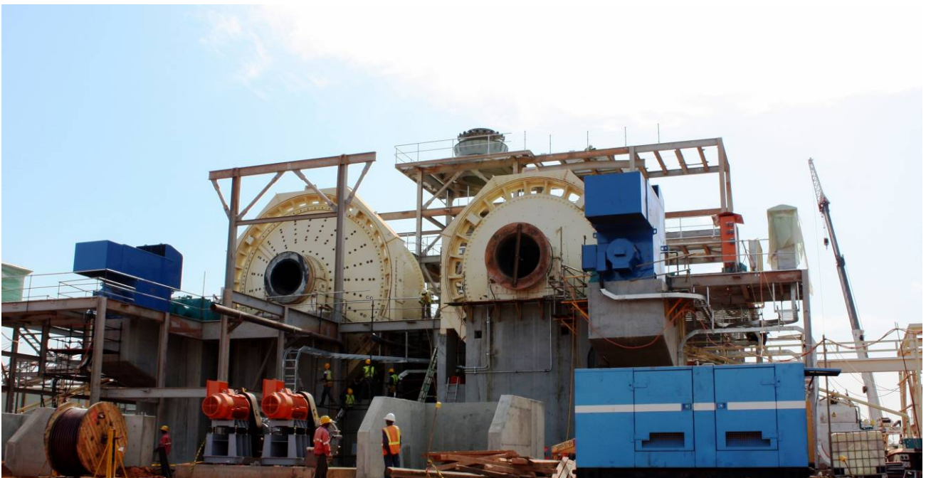
Grinding mills nearing completion
