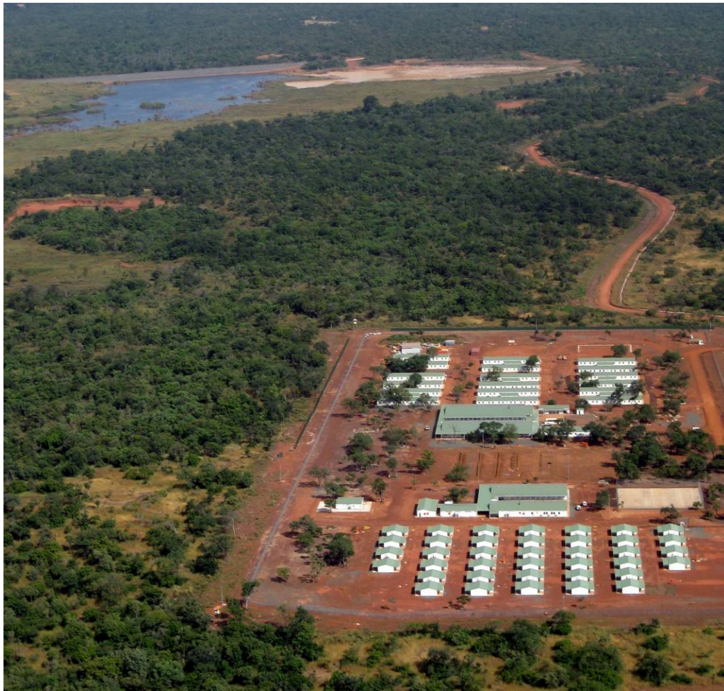
Sabodala accommodation village with main water storage dam in background
