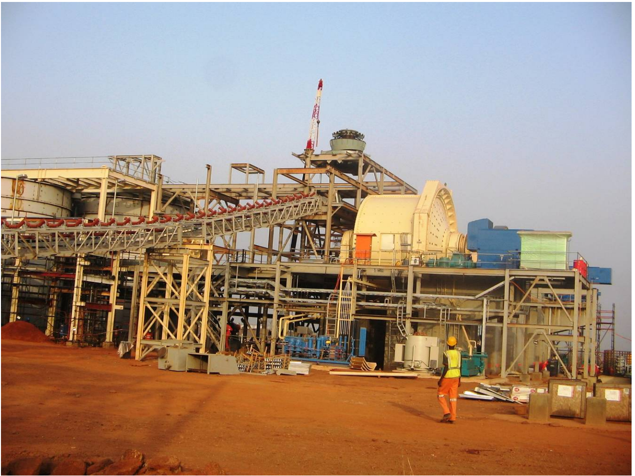
Close up of the main feed conveyor, CIL tanks and SAG and Ball mill
