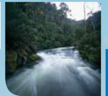
Bogong Hydro-Electric Power Station
