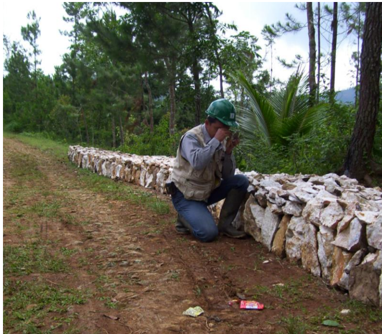
Checking gold-mineralised quartz-breccia vein boulders from Bonang vein used for road aggregate, Kojan Prospect
