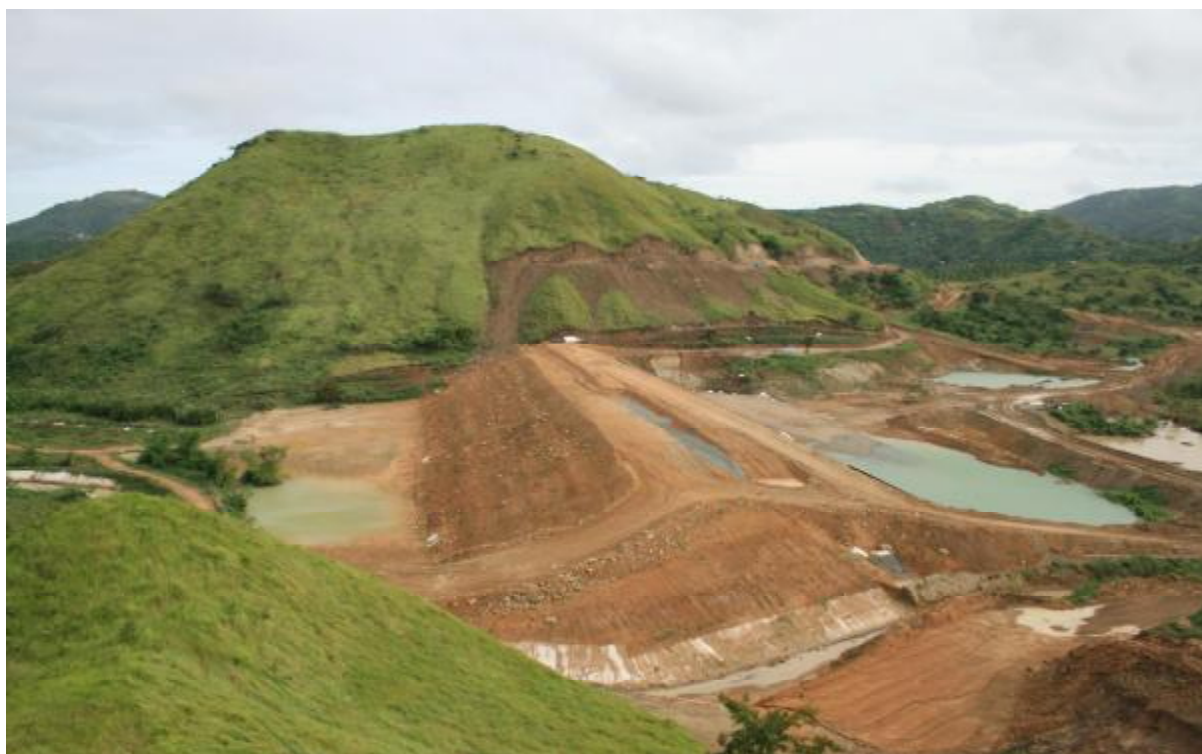
Tailings Dam as at 16 January 2009
