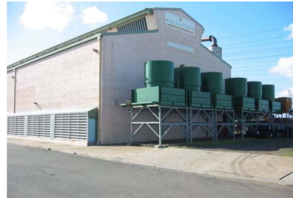
Existing generating station, Sunshine
