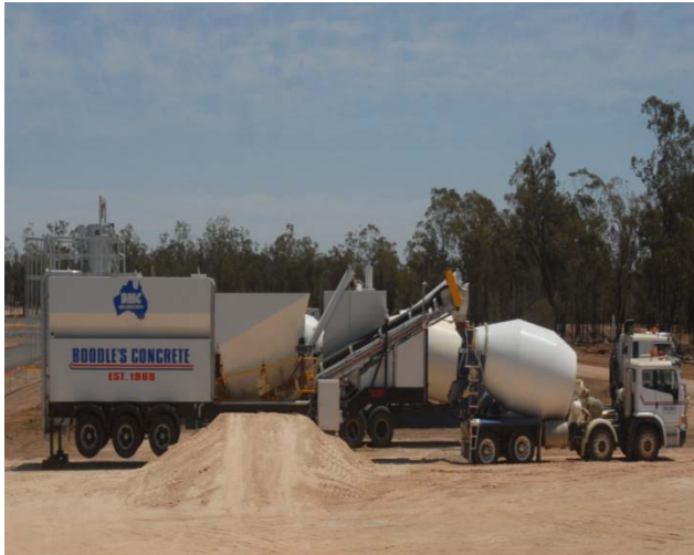
Foundations being laid
