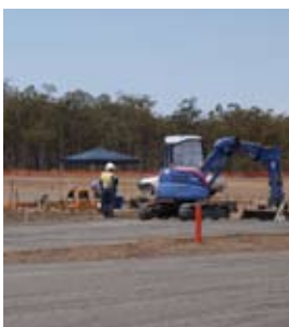
Foundations being laid
