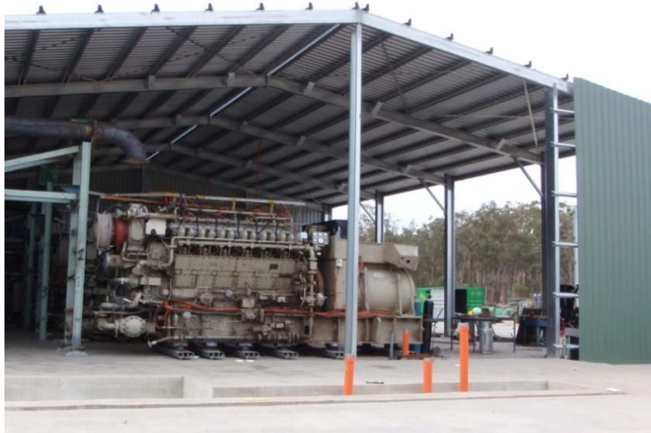
November 2009 – Construction of Gas Engine hall at Bloodwood Creek
