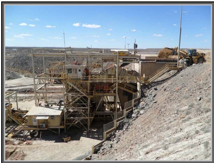
Side view of BGSM primary crusher being loaded with CRE ore
