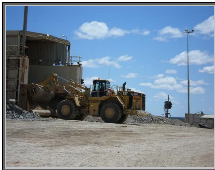
Barrick loading Crescent ore into the BGSM hopper
