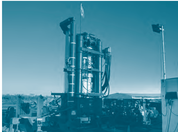
Raise Bore – Drilling Ventilation Shaft Pilot Hole
