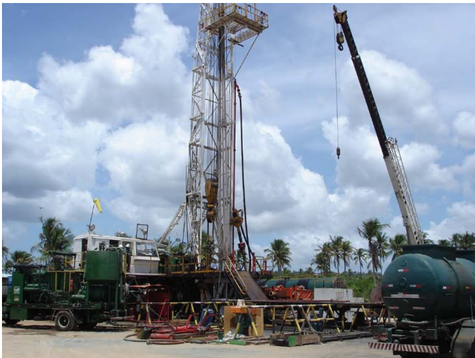
Figure 1 – Flow testing of the PACA 2 Discovery
