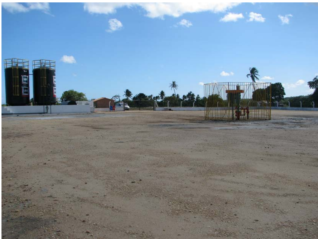
Figure 2 – Production testing facilities at PACA 1
