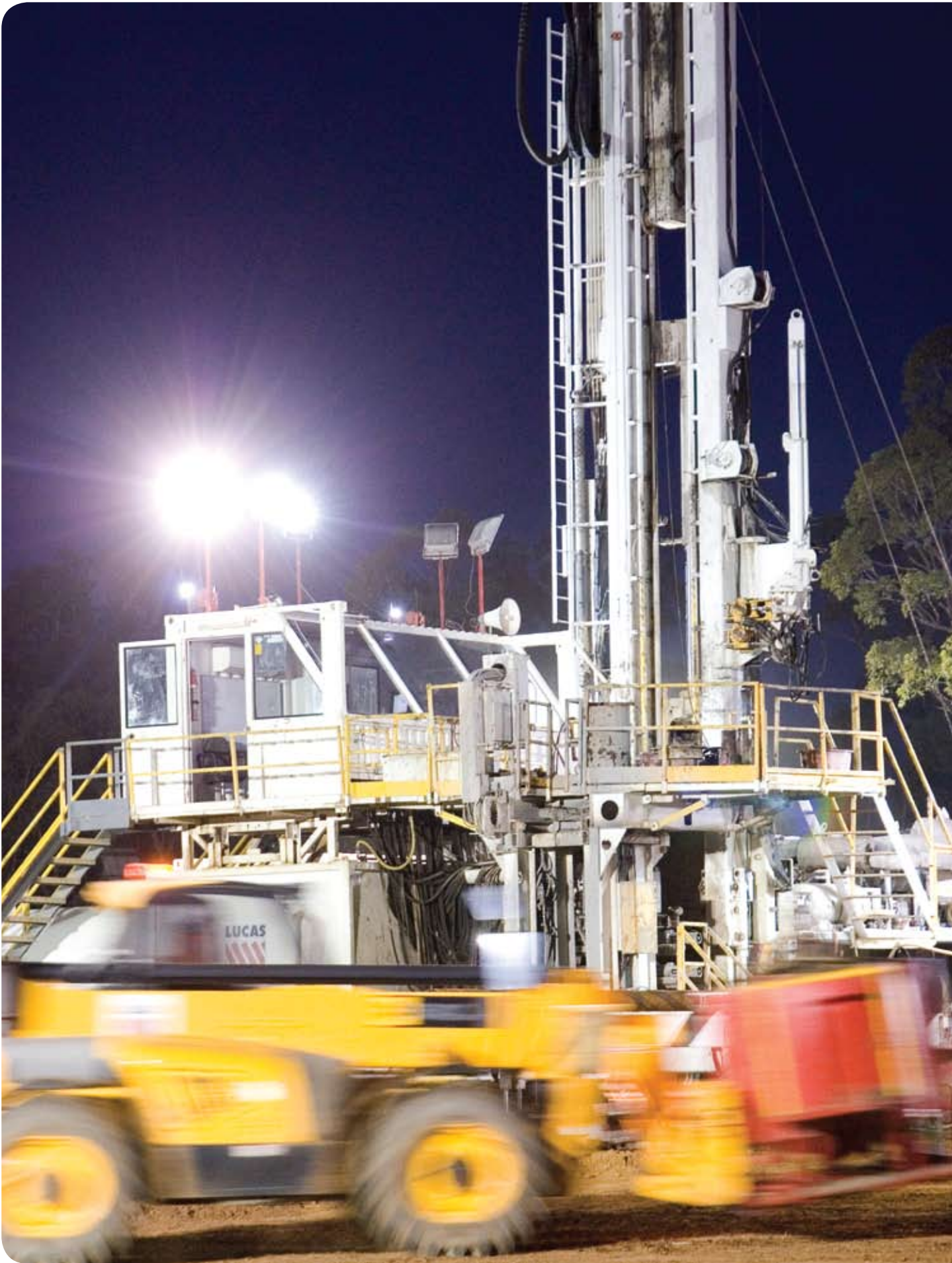
Lucas Rig 26 on 24 hour operations
