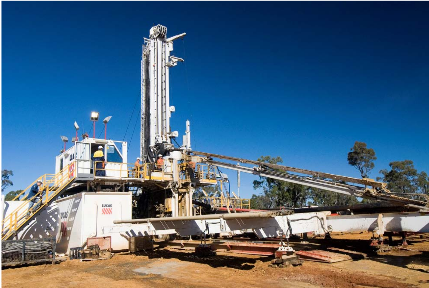
Schramm TXD Drilling Rig on site at Narrabri
