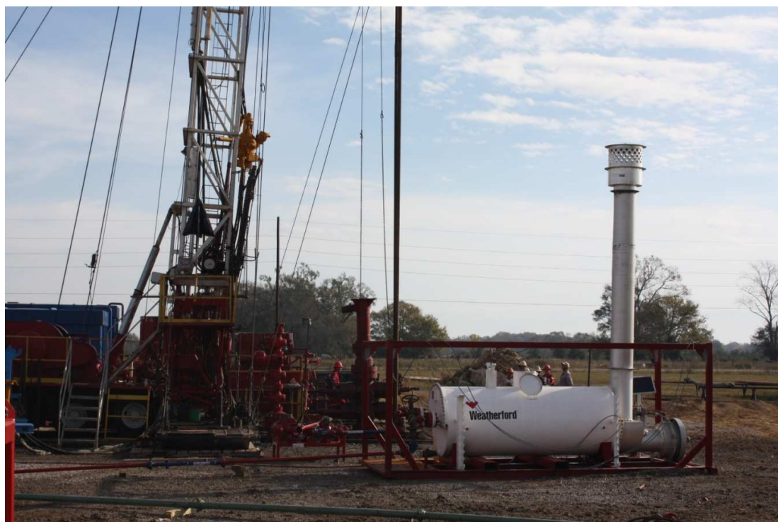
Perforation of the HM Brian No.1 well and associated testing equipment supplied by Weatherford
