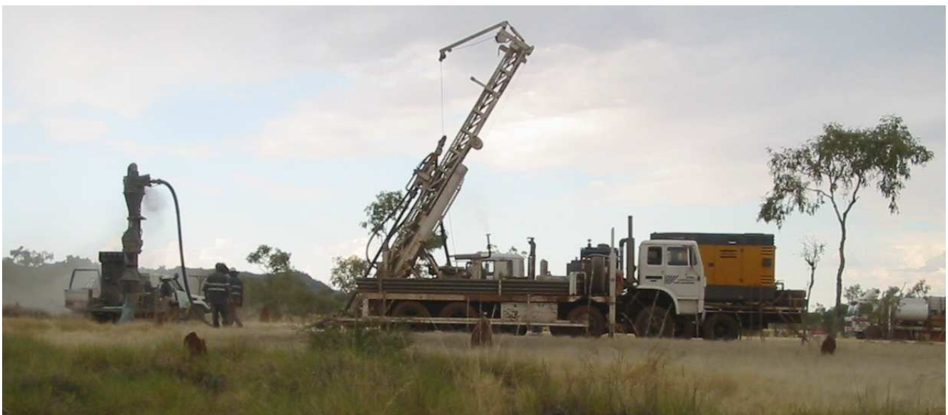
Drilling in progress at the Tambourine prospect.
