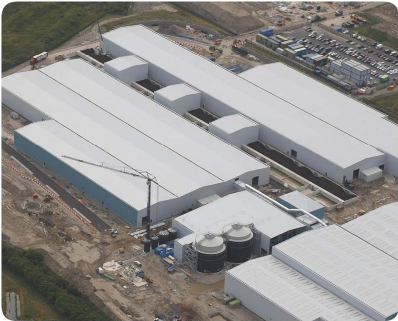
Construction at Lancashire Waste Project's Thornton site
