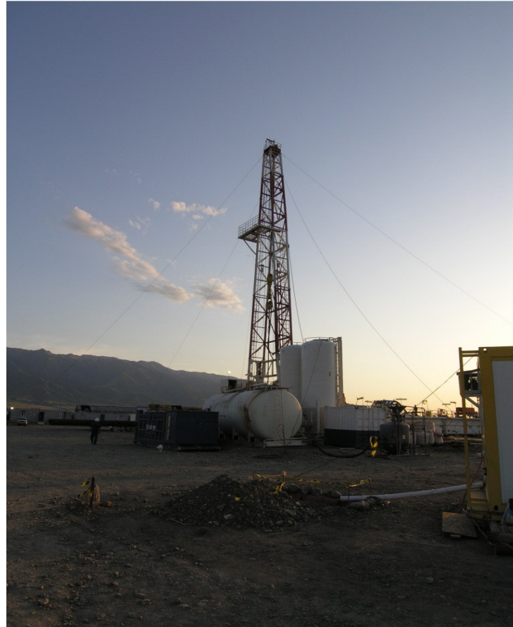
Figure 5: drill mobilised ahead of drilling
