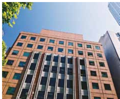
QBE HOUSE 628 Bourke Street, Melbourne, VIC
