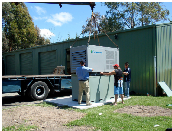
Skywater 300 display unit being installed at Narre Warren
