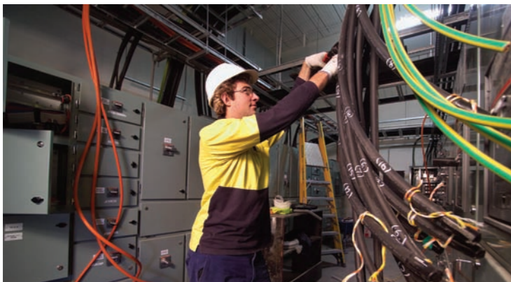
Installation of sub-mains cables to main switchboard
