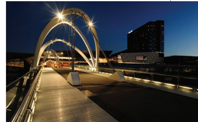
Intelligent lighting control solution at Yarra Footbridge
