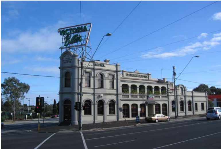
Elsternwick Hotel, Melbourne, VIC
