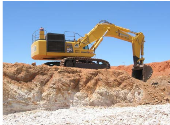
Free Dig Excavating of Overlying Waste Rocks
