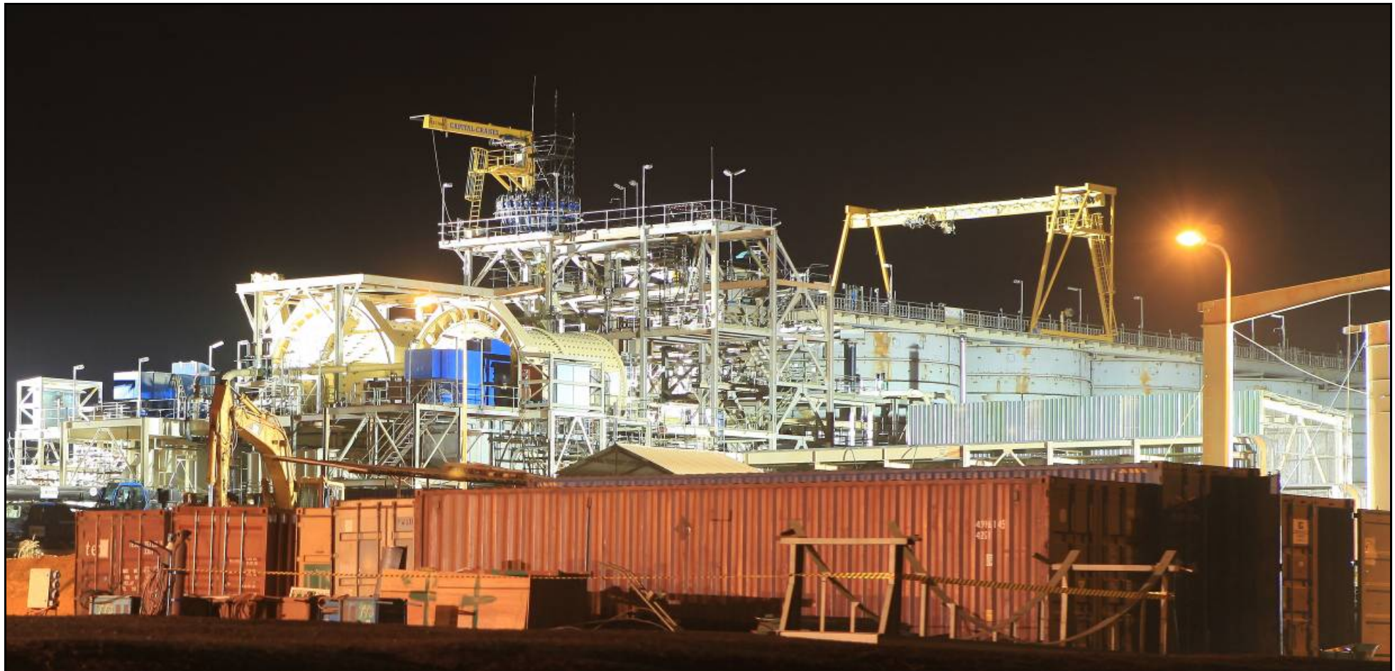
Plant showing SAG and ball mills in yellow and CIL tanks in background
