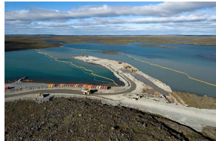
Cofferdam construction at Meadowbank Gold project, Nunavut, Canada
