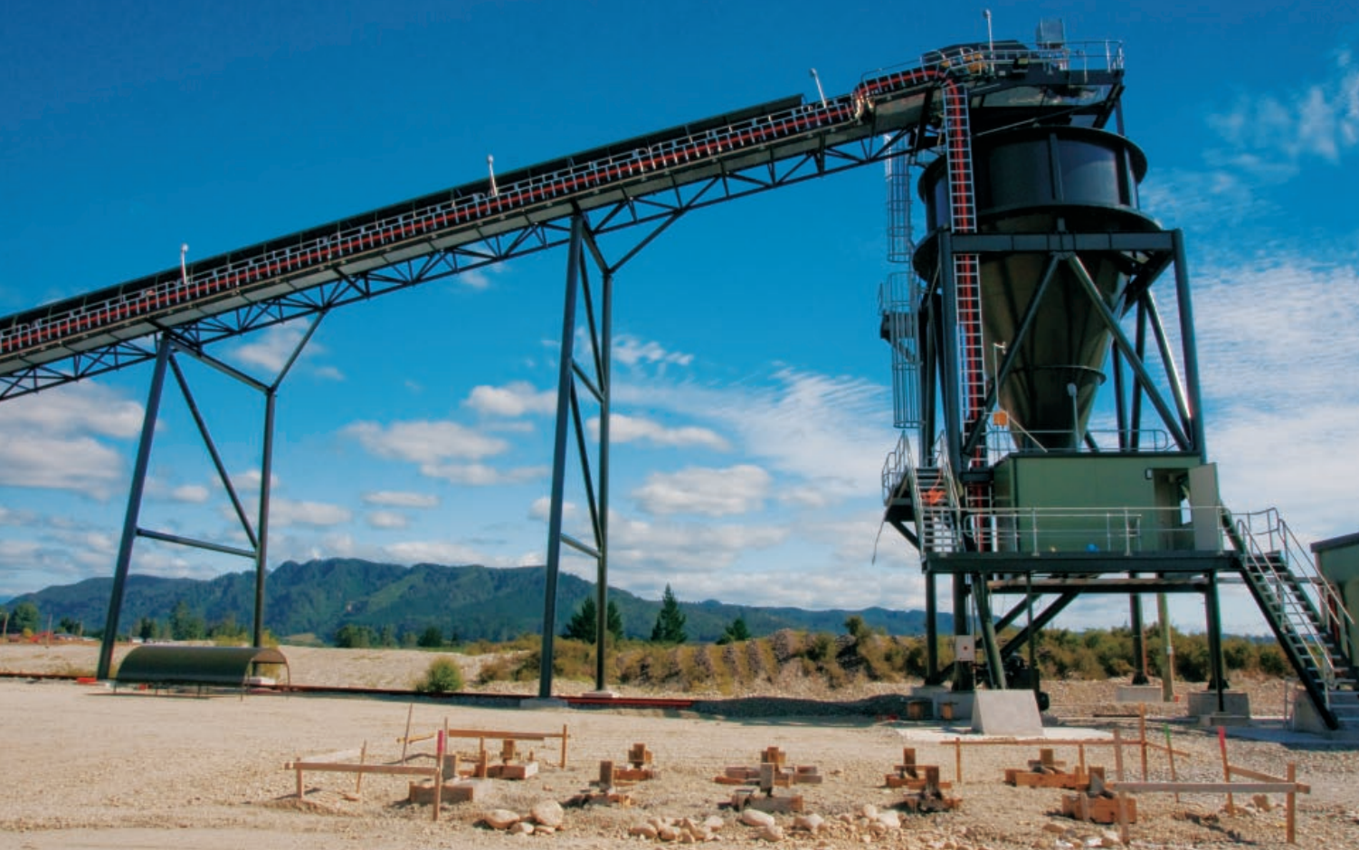
Ikamatua rail loadout facility
