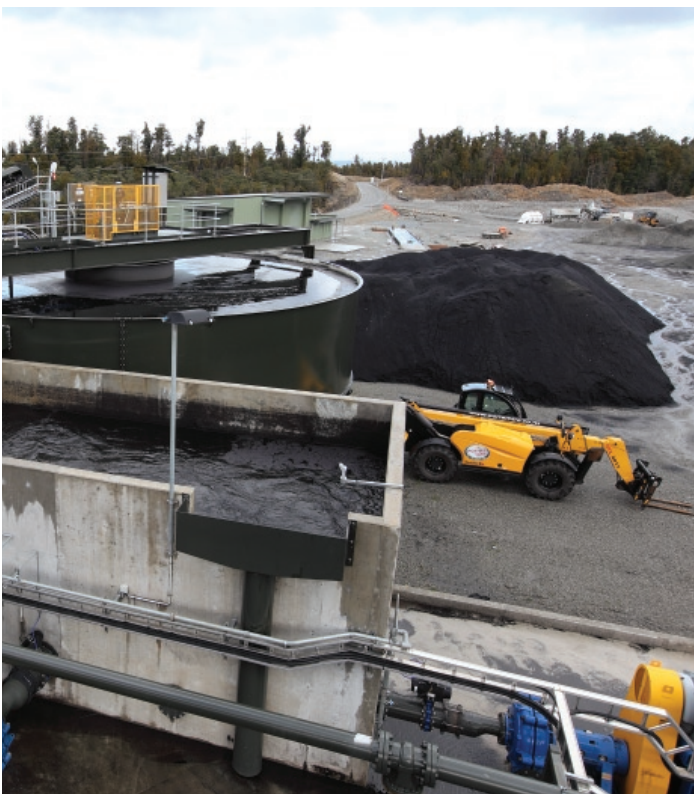
Pike River coal preparation plant
