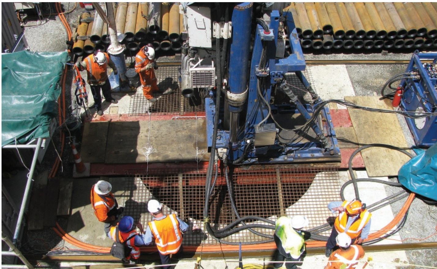
Raise-boring the main ventilation shaft
