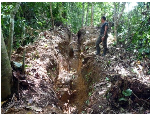
Trenching at Jelatang
