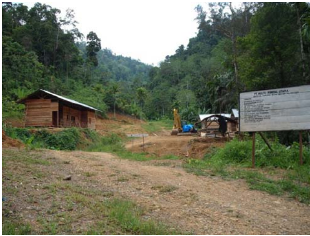
Camp construction at Pinang-Pinang
