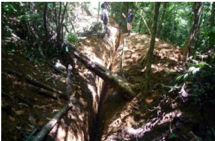
Trenching at Nilam
