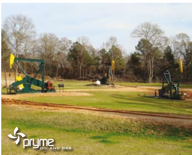
Wells located in Routh Point Field, LaSalle Parish
