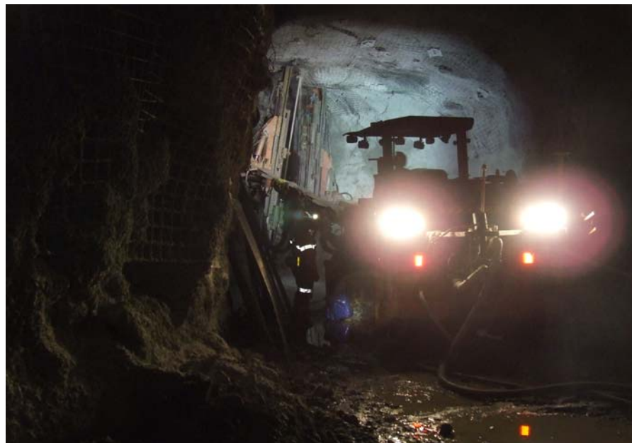
Twin Boom Jumbo underground at Wattle Dam
