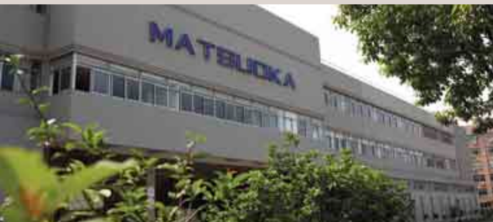
Matsuoka headquarters Xiaoshan National Economic Development Zone, Hangzhou, China.
