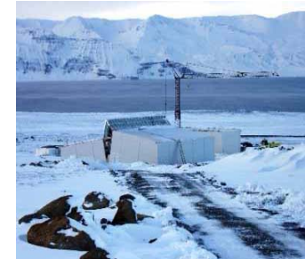
Geothermal Plant (Iceland)
