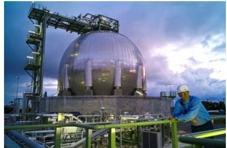
Hiteshkumar Raval at the LNG plant in Kwinana, WA August 08
