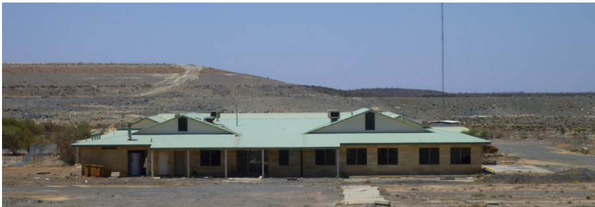
Central Murchison Gold Project Site Office
