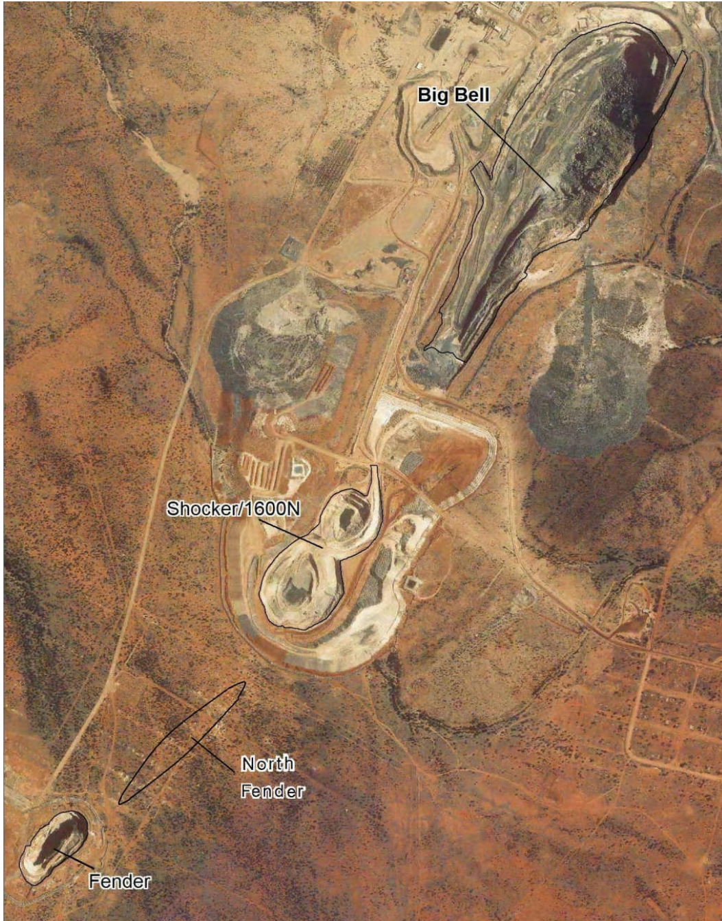
Aerial photo of Murchison Bell Mining Centre showing the location of the North Fender Prospect - Total Identified Mineral Resource Estimate (JORC) of 51,257 ounces
