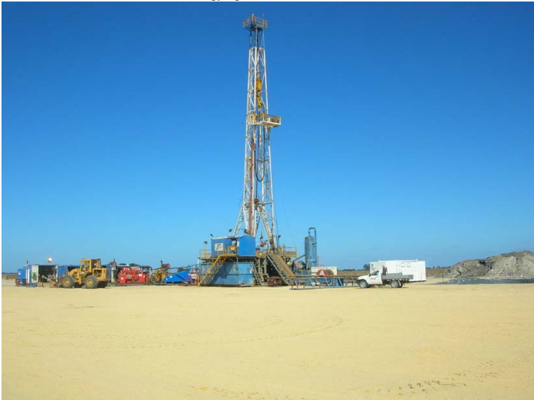
Hunt Energy rig on the Hollick-1 well site:
