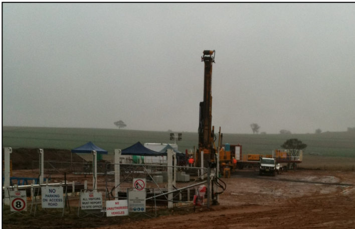
Turill-1 drill site
