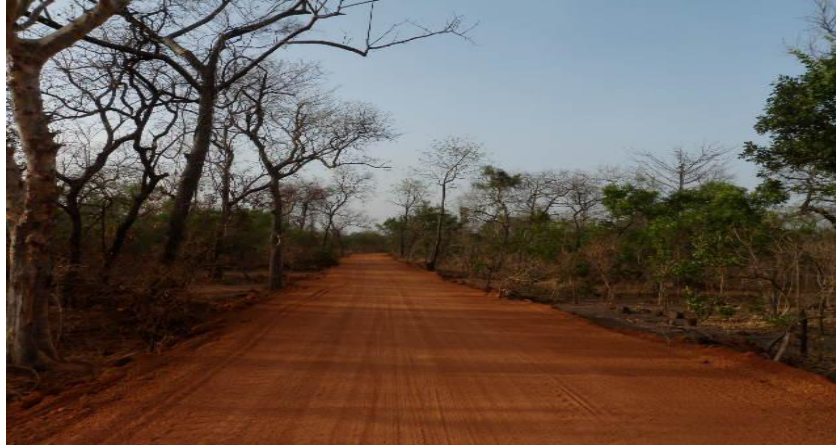
Figure 5 - A section of the new Douta – Makabingui road
