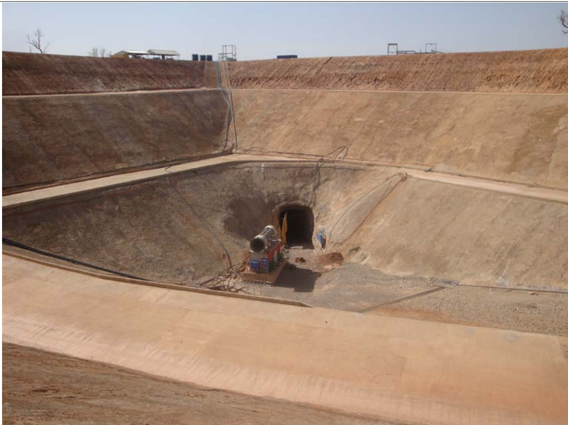
Box-cut and portal Photo taken: 4/2/2010
