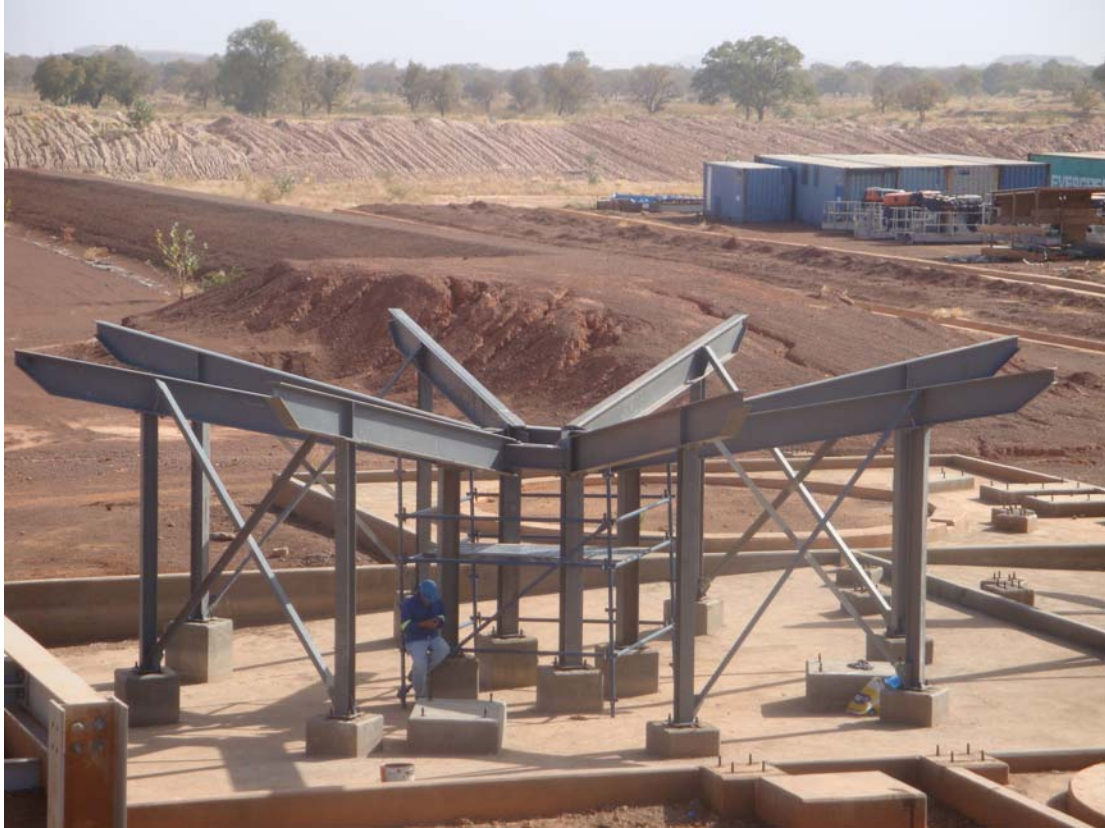
Foundations and Steel Framework for concentrate thickener tank Photo taken: 6/2/2010
