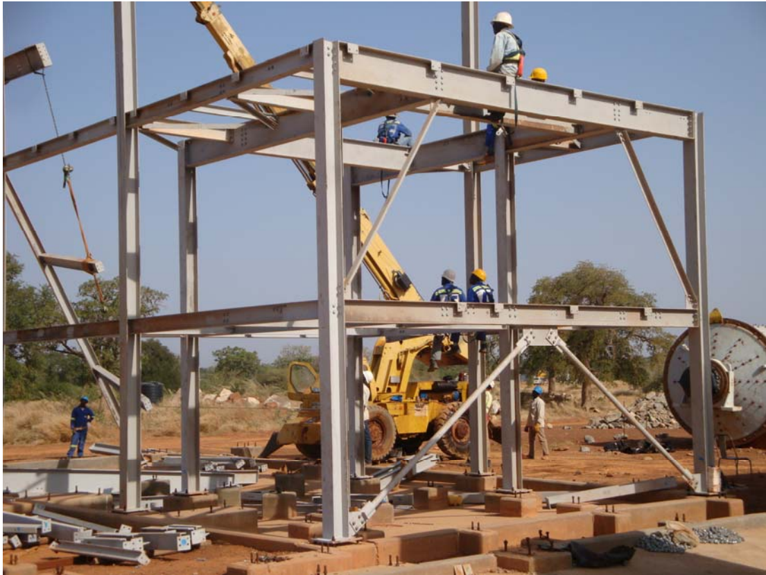
Assembly of steel work for process plant Photo taken: 4/2/2010
