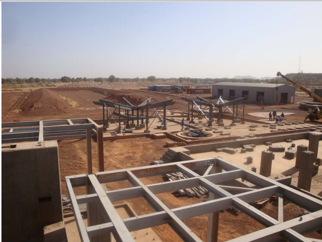
On-site construction continues Photo taken: 6/2/2010
