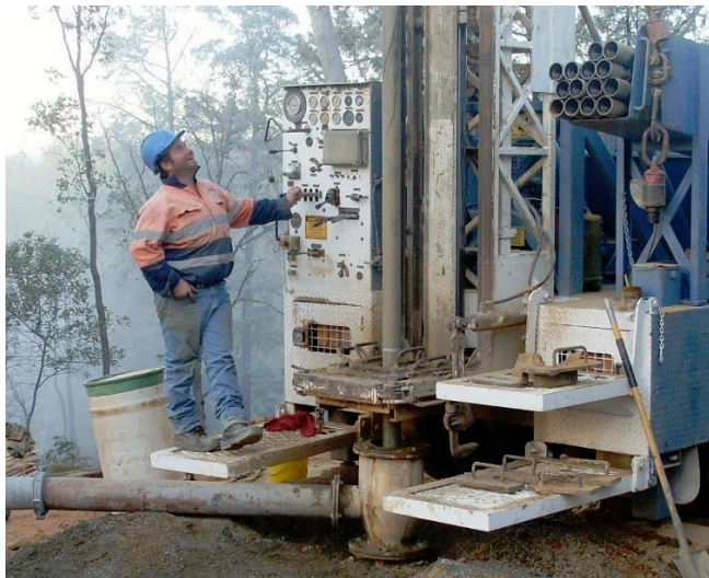
Ten inch Percussion Drilling in Progress
