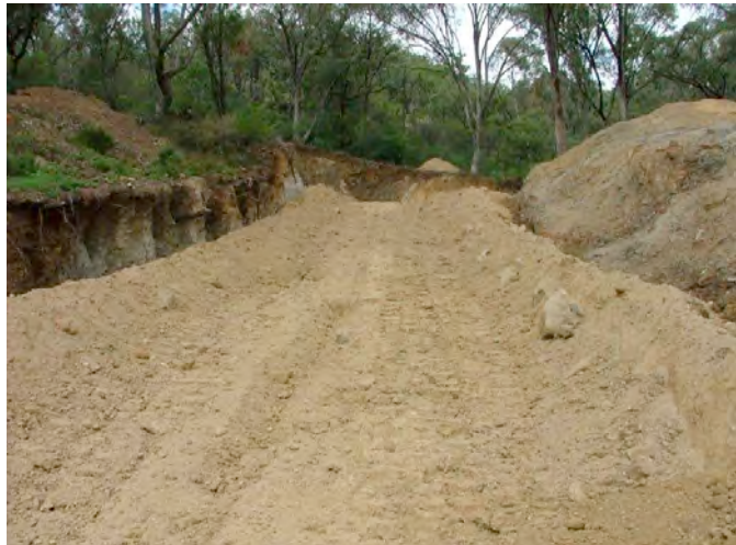
Cluff's restoration of Upper Four Mile area during September 2010
