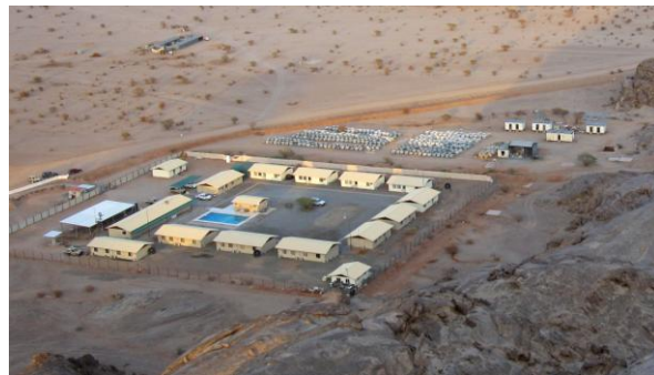
Figure 2: Jabal Sayid camp refurbishment
