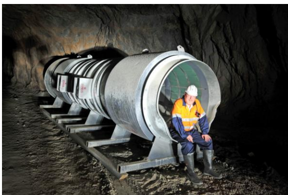
Figure 1: Underground decline refurbishment
