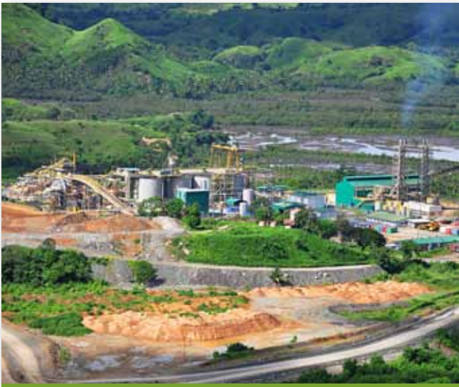
The Masbate Gold Project
