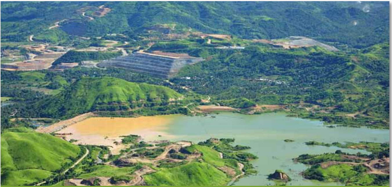
Tailings Storage Facility
