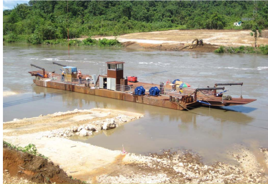
Ferry Assembly Nearing Completion – Winches Positioned
