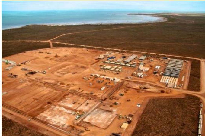
Fly camp featured in the top right corner of the construction village area in this picture
