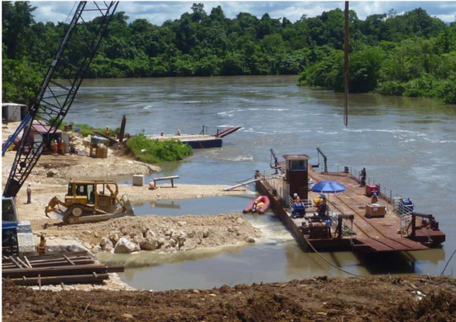
Construction of Ferry Access Track
