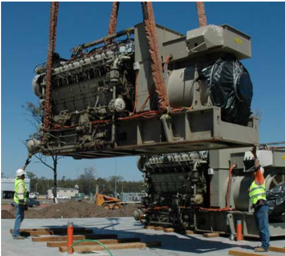
Gas engines being positioned On site - October
