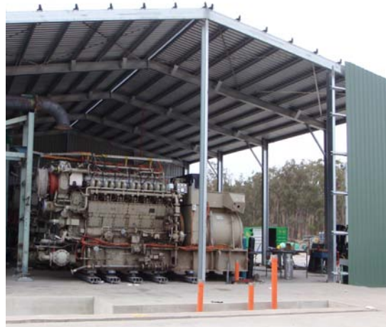
Power station buildings Constructed - December
