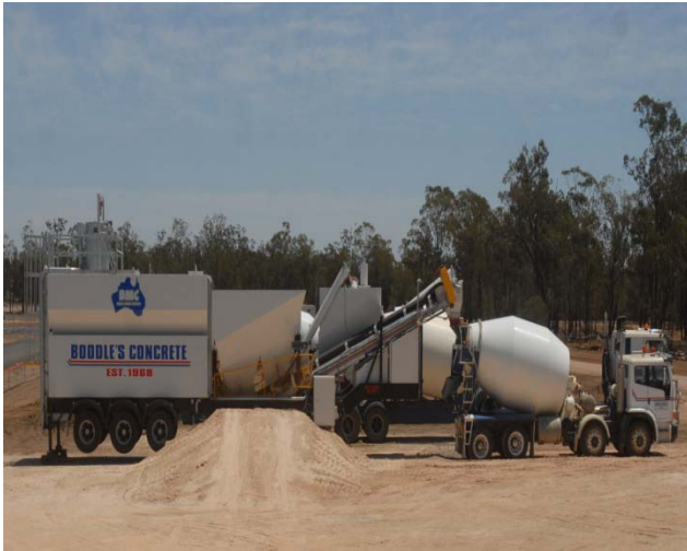
Foundations being laid
