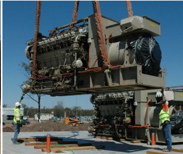
Gas engines being positioned on site
