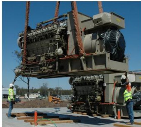
Gas engines being positioned On site - October
