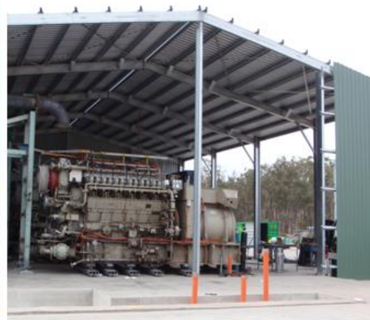
Power station buildings Constructed - December
