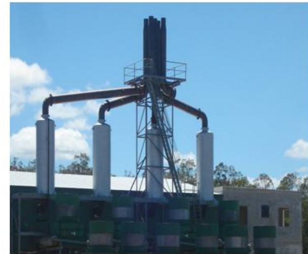
External equipment in place - January
